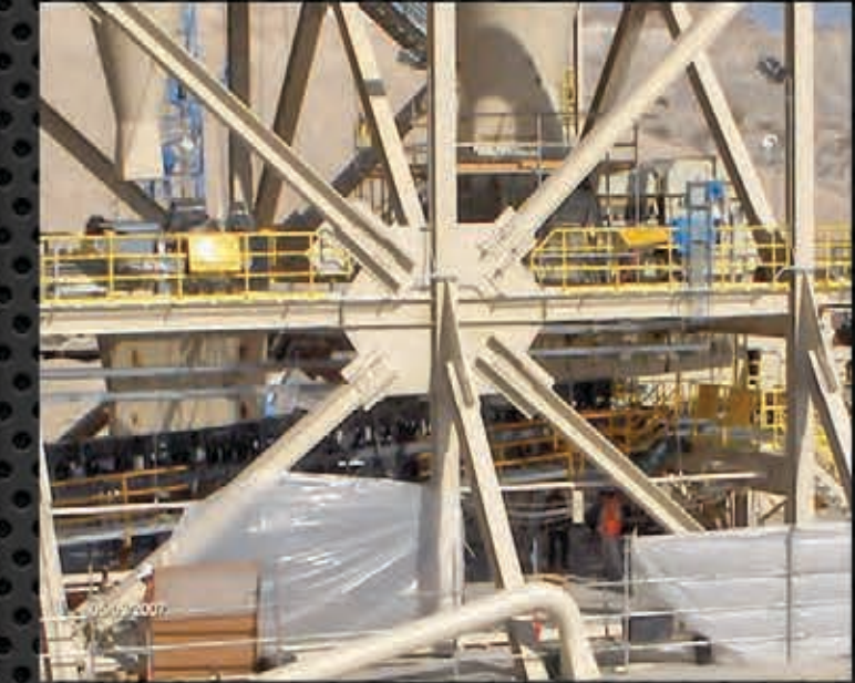
Oro Grande Cement Plant Victorville, CA
