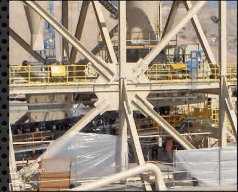
Oro Grande Cement Plant Victorville, CA
